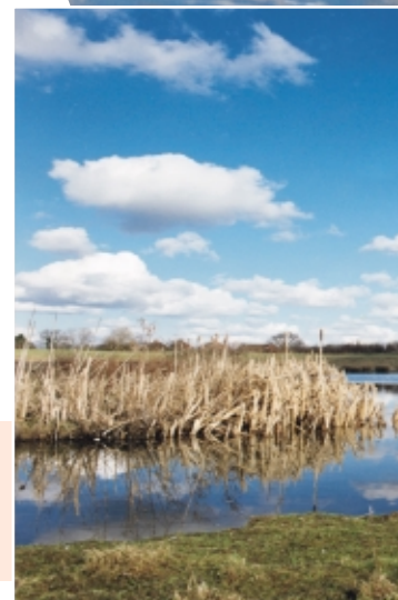
HUM Storm Water Lagoon
