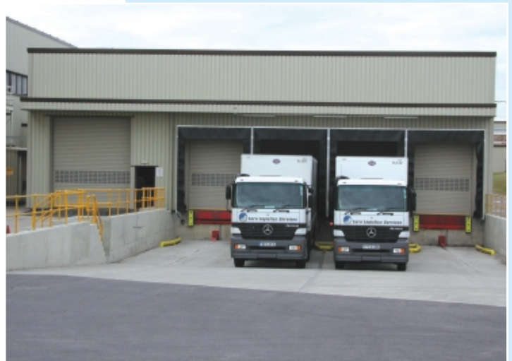
Material Logistics Building (ML)
