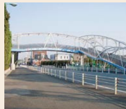
Newly erected pedestrian overpass at the factory entrance
