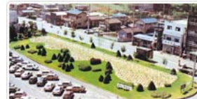
Area around the front of the Sayama Plant at Saitama Factory when the Community Forest initiatives were launched in 1977; seedlings are being planted in the areas covered by white-looking straw.
