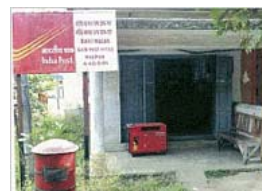
An EXK2800 being used as a computer backup power supply in India
