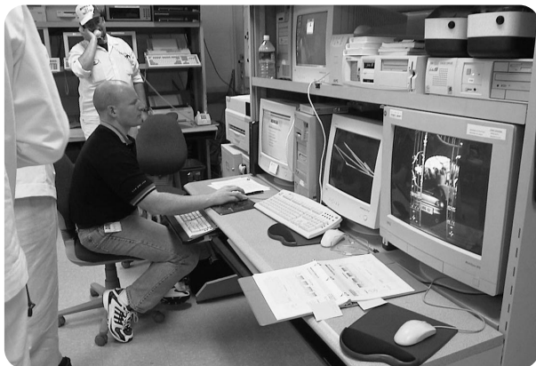
Computer control office
