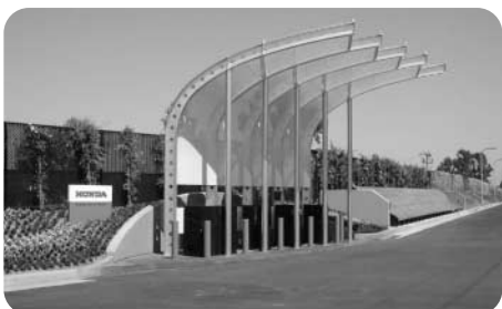
Hydrogen manufacturing and supply station
