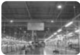
Before the installation of skylights
