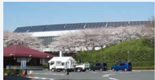
Solar power facilities
