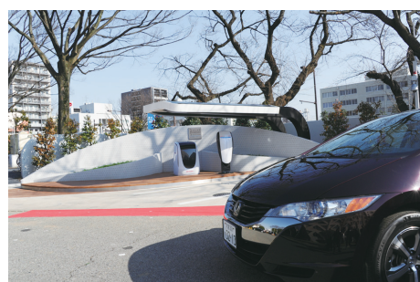
FCX Clarity and solar hydrogen station installed at the Saitama Prefectural Office
