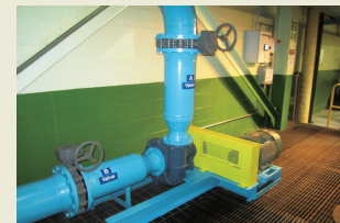
Newly introduced hydropower system
