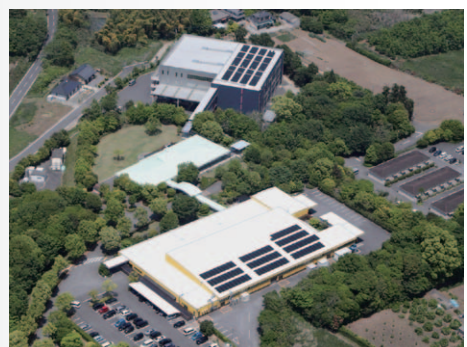
Solar panels installed at Honda Sun
