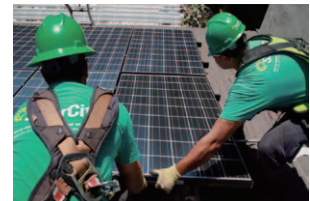
A solar power system being installed at a customer's home
