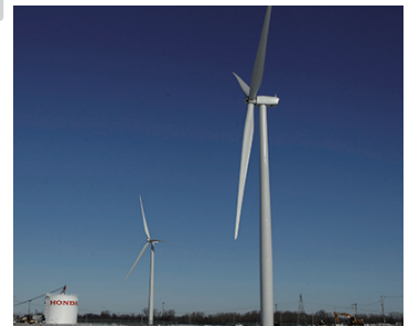
Two 1.7 MW wind turbines provide about 10% of the plant's electrical needs
