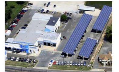
Rossi Honda's solar PV system
