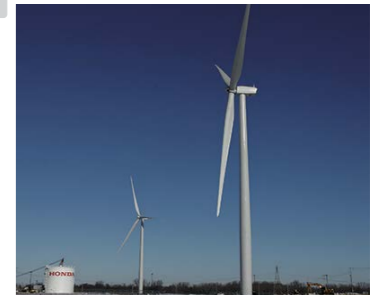
Two 1.7 MW wind turbines provide about 10% of the plant's electrical needs
