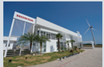
Honda Energy do Brasil Ltda. has nine wind power turbines
