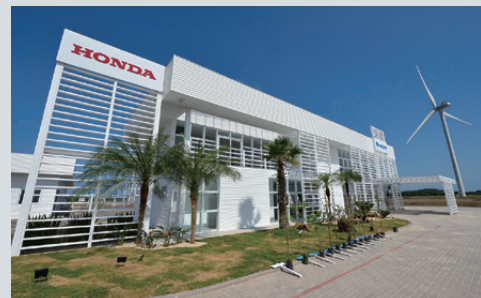
Honda Energy do Brasil Ltda. has nine wind power turbines
